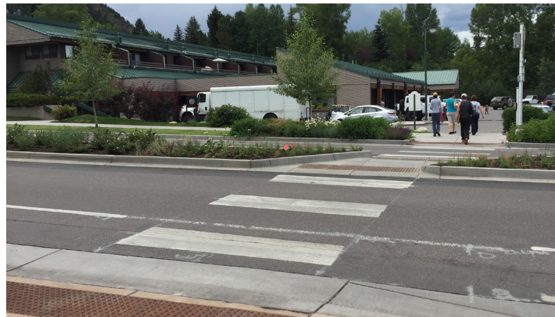
Pedestrian refuge islands help to improve safety for crossing pedestrians, especially on multilane roadways (Image: Aspen, CO)
