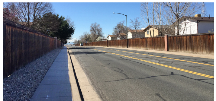
Many streets in Westminster are flanked by long walls of fencing which detract from the pedestrian experience (Image: Westminster Blvd north of 92nd Ave).
