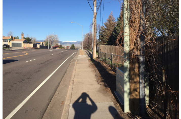
Sidewalks placed along high-volume, high-speed roads without buffers are uncomfortable to walk along (Image: 92nd Ave West of Raleigh St).
