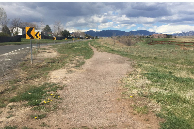
Informal paths have been created where there is demand for a sidewalk, but where no sidewalk exists (Image: W 108th Ave west of Westmoor Dr).
