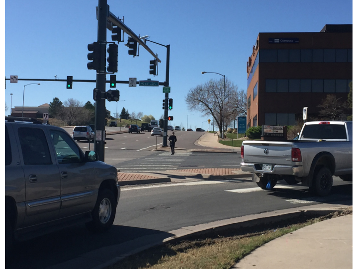
Most major intersections in Westminster have right turn slip lanes that channelize right-turning vehicles, which increases intersection efficiency from a vehicular standpoint but also can make crossing intersections more stressful for pedestrians (Image: Sheridan Blvd and 92nd Ave).
