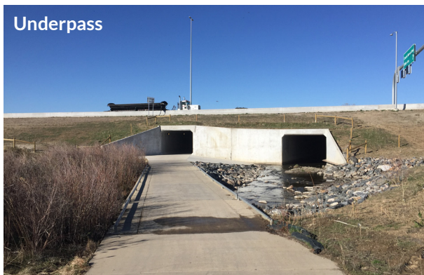
Image: Big Dry Creek underpass at US 36 and 103rd Ave
